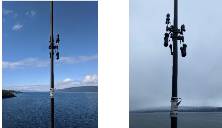
Figure 1: The left picture shows a hanger with two Stockbridge dampers, while the right image shows a hanger with three Stockbridge dampers
